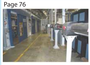
Page 76 Beam Pipes
