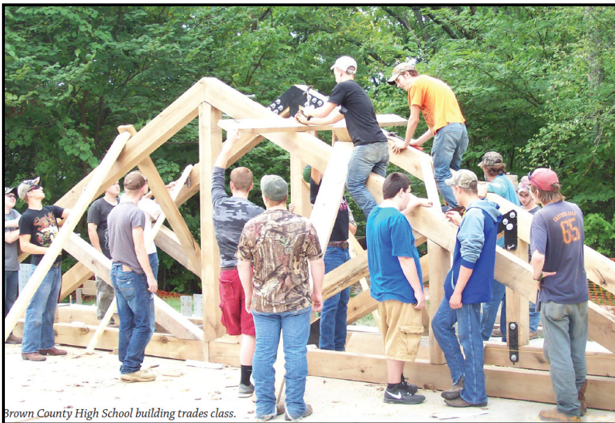
Brown County High School building trades class.
