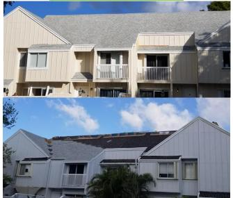
Ridge vents will be eliminated and replaced with additional passive venting. Existing gutters will be removed and replaced at the Association's expense. Owners are responsible for the cost of replacing any rotten plywood on their roof and fascia. Some sections of screen (not the frame) may need to be removed to provide ladder access as the roofers are working. Any existing screens removed will be replaced at the Association's Expense.
