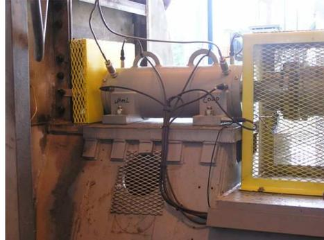
**Figure 35. Photo of Newly Installed One Piece Bearing Housing With Accelerometers and Temperature Sensors Installed.**
