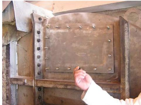
**Figure 37. Photo of Modified Fan Housing to Install Access Panel for In-Place Balancing & Inspection.**
