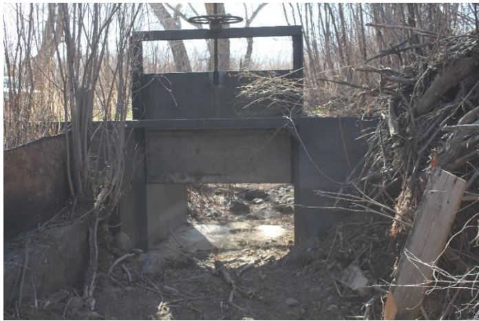
Headgate looking downstream
