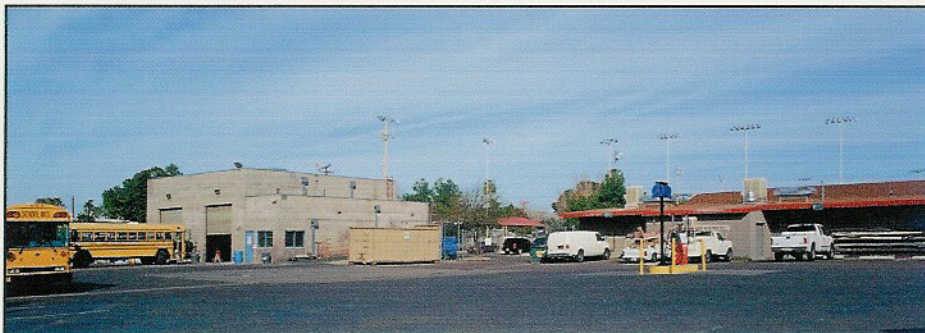
Madison School Bus Facility Phoenix, Arizona
