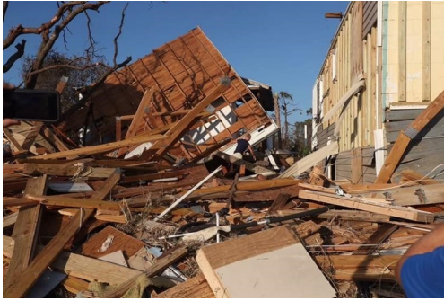
Two photos of the general devastation.
