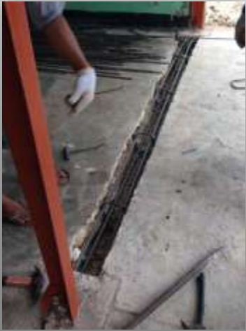
Plinth beam construction using rebar
