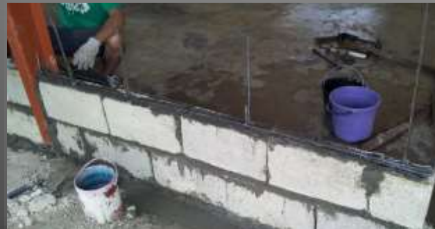
Connection of the horizontal rebar onto vertical rebar
