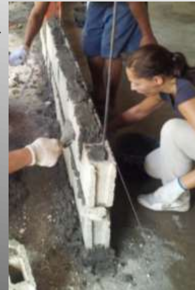
Hollow blocks filled with concrete.
