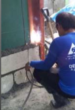
Welding of horizontal rebar to steel column
