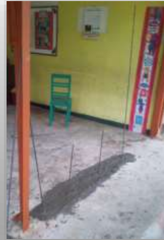
Plinth beam completion
