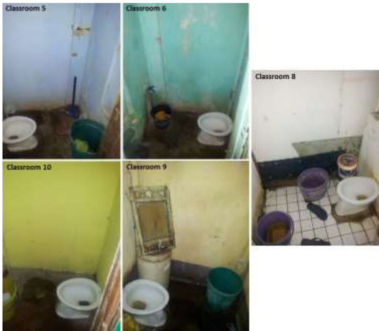
Comfort Rooms identified for refurbishment.
