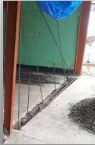
Vertical rebar for the concrete hollow block walls
