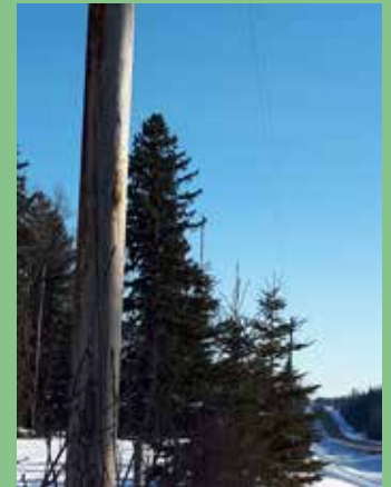
But...they grow – into the powerline see upper right.
