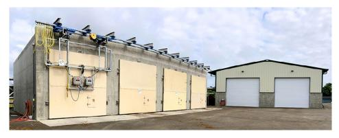
The City of Long Beach (CA) composts biosolids in aerated tunnels (above left) supplied by Engineered Compost Systems.
