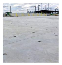
Newly built sparger type floor for the positive aeration mass bed used for curing (foreground). Active composting bunkers and preprocessing building (on far right) are in the background.
