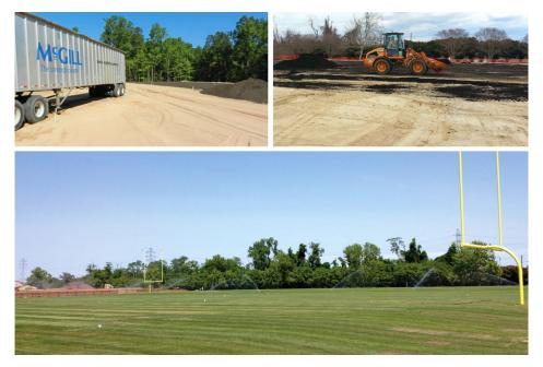
McGill SoilBuilder Premium Compost was used in construction of practice training fields for the Washington NFL team and the University of North Carolina-Charlotte. The fields were leveled, compost was spread and incorporated into the soil, and sod was laid on top.
