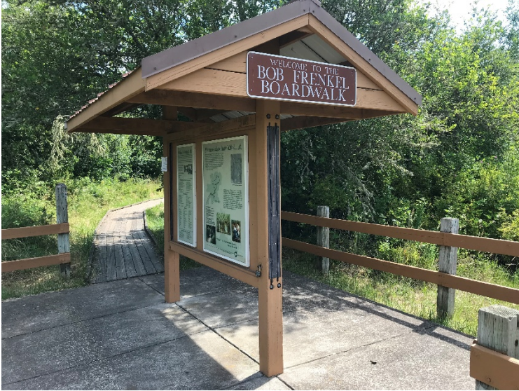
Existing kiosk at the Jackson-Frazier Wetland
