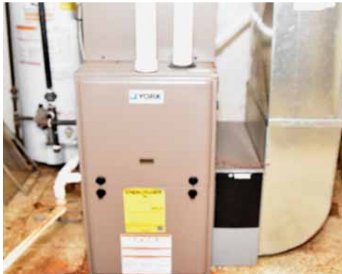
Furnace/Water Heater
