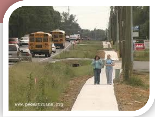
In high traffic areas, sidewalks are feasible when placed away from the road or when some other safety barrier is implemented.
