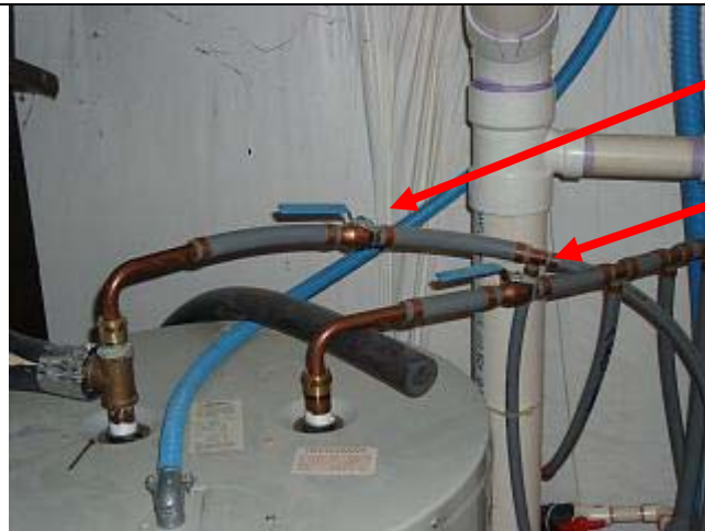
Water shutoff Outflow Intake
