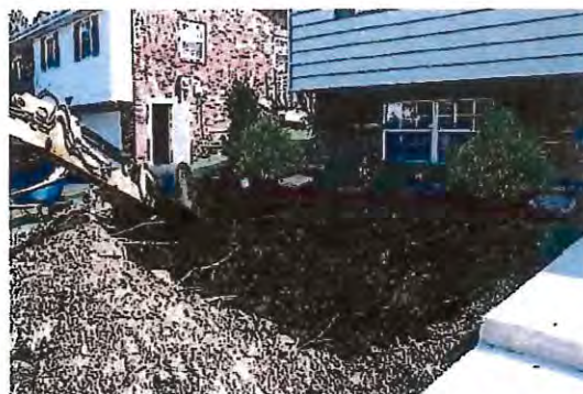
Excavate rain garden at least 10' from foundation
