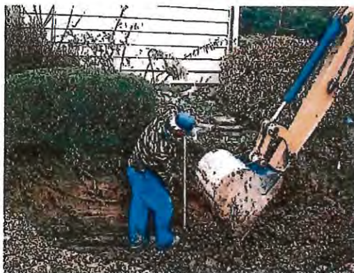
Excavate a drywell at least 10' from foundation
