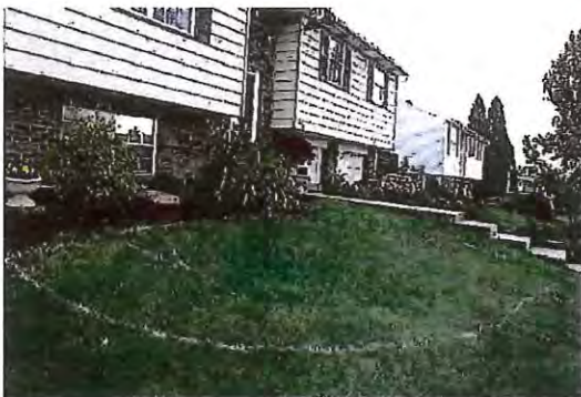
Mark rain garden location to avoid utilities
