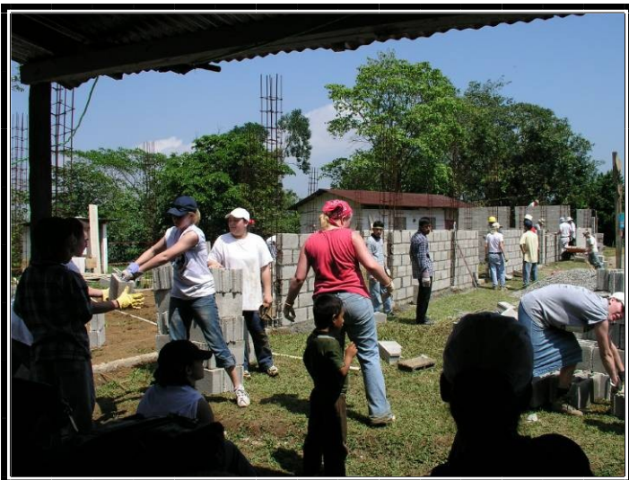
Construction crew hard at work on new classrooms
