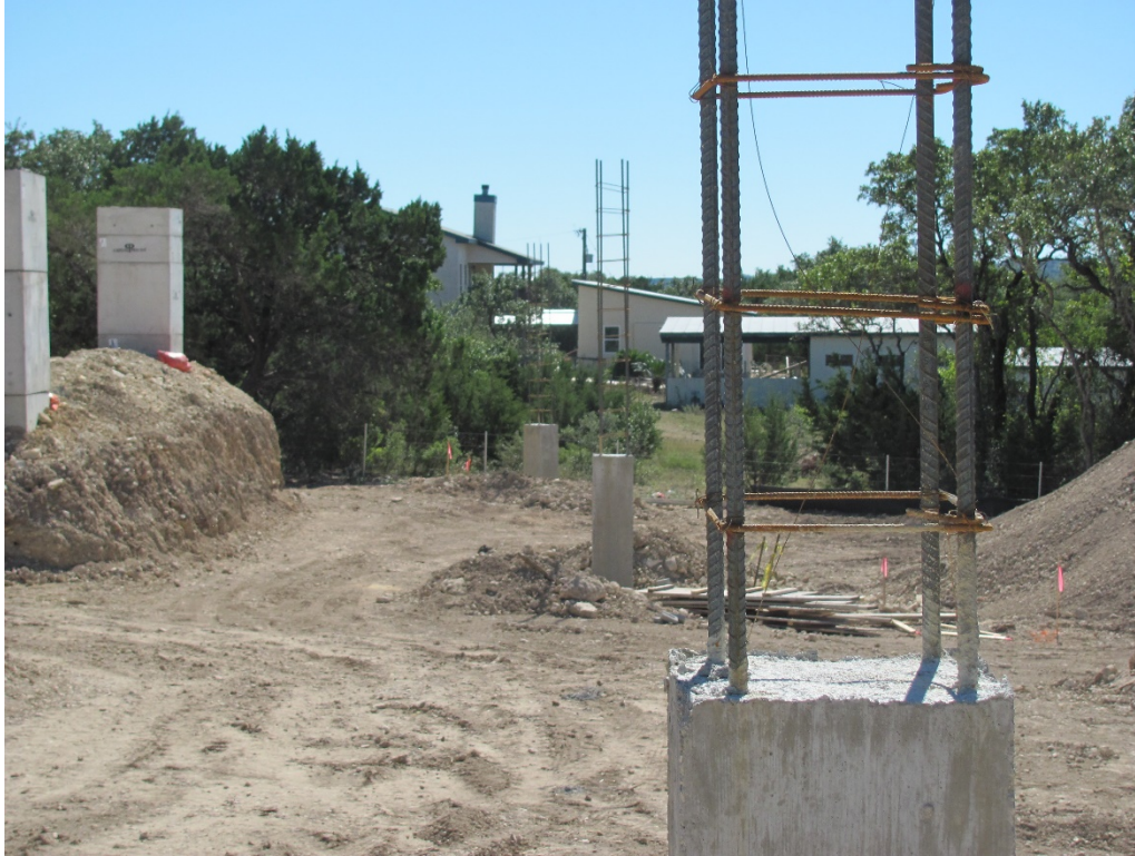
EXHIBIT 11 – CONCRETE: LIGHT STANDARDS POURED COLUMNS 10.28.20
