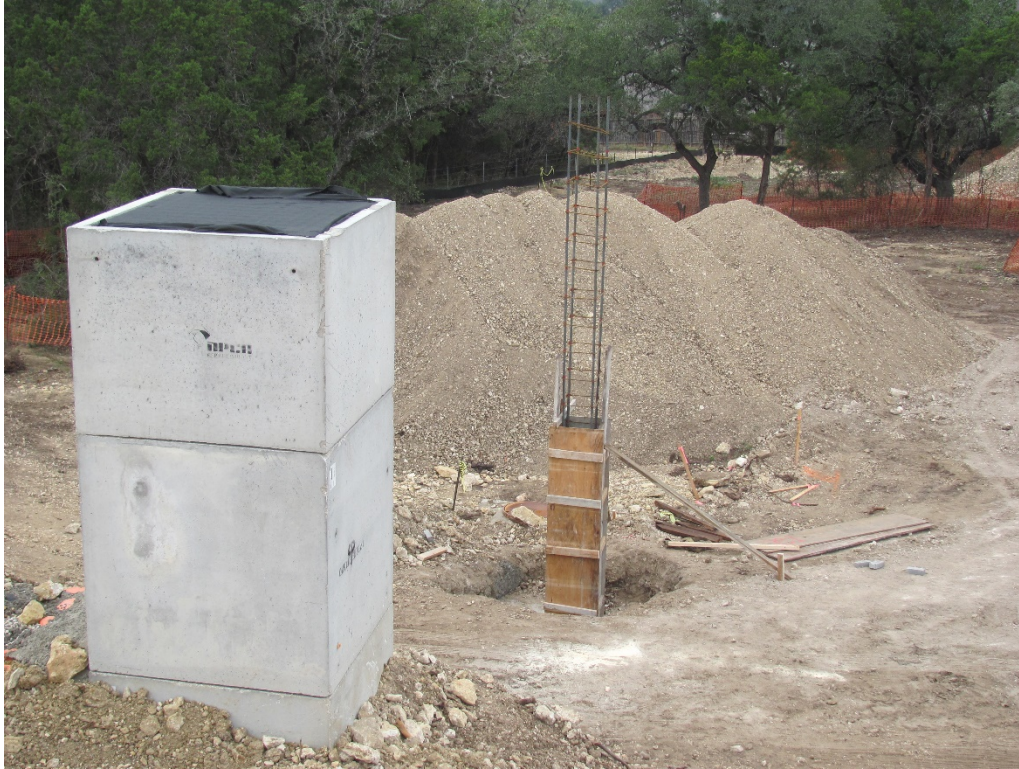
EXHIBIT 9 – CONCRETE: FORM LIGHT STANDARD 10.26.20
