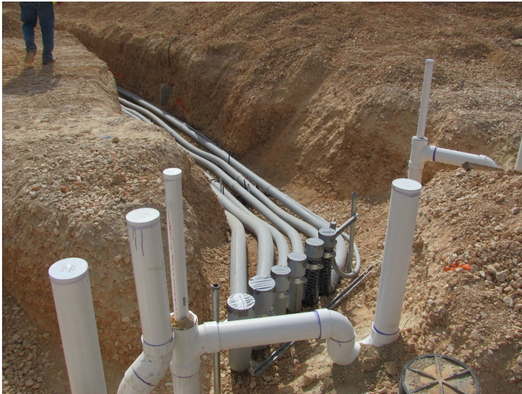
EXHIBIT 4 – ELECTRICIAN: BUILDING PAD CONDUIT INSTALL 10.09.20
