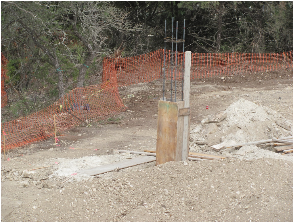
EXHIBIT 8 – CONCRETE: FORM LIGHT STANDARD 10.23.20
