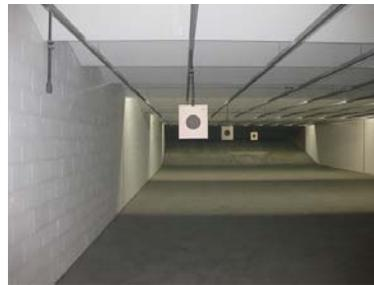
The closest target is too close. If you look 'through' the target bullseye, you can see that the bullets would hit the ceiling baffles instead of entering the trap system 'funnel'. This target is not safe to shoot at and may cause unintended damage.
