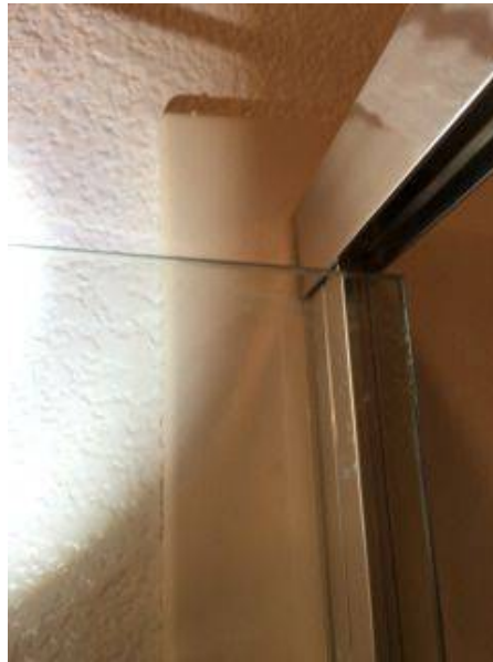
Photo 29-2 No Tempered Glass Picture 2
