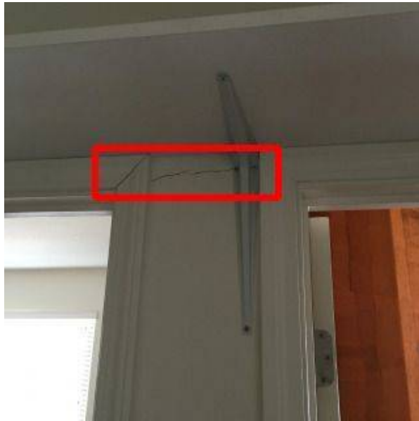
Photo 34-2 Drywall Crack 3
