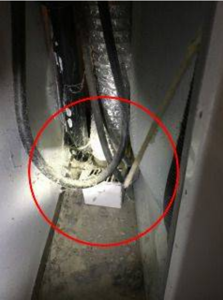
Photo 11-1 Garage Dryer Vent Duct
