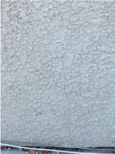
Photo 4-3 Stucco Crack 4
