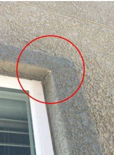
Photo 4-1 Stucco Crack
