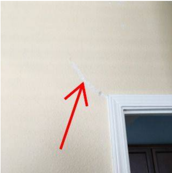
Photo 34-1 Drywall Crack 1
