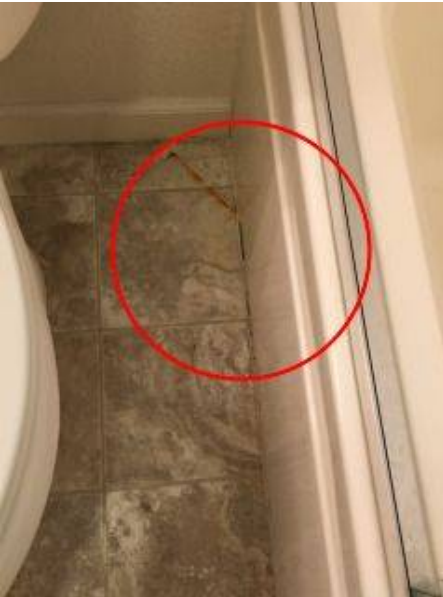
Photo 32-1 Caulk Repair
