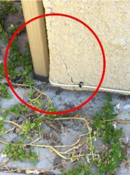
Photo 3-1 Stucco Crack 2
