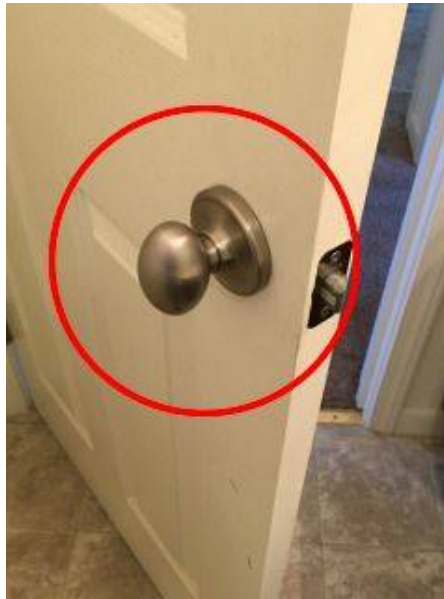
Photo 35-2 No Bathroom Door Lock
