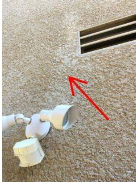
Photo 4-4 Stucco Crack 5
