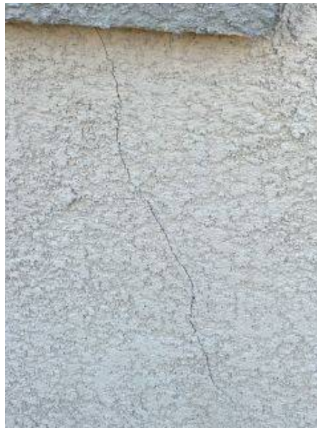
Photo 4-2 Stucco Crack 3
