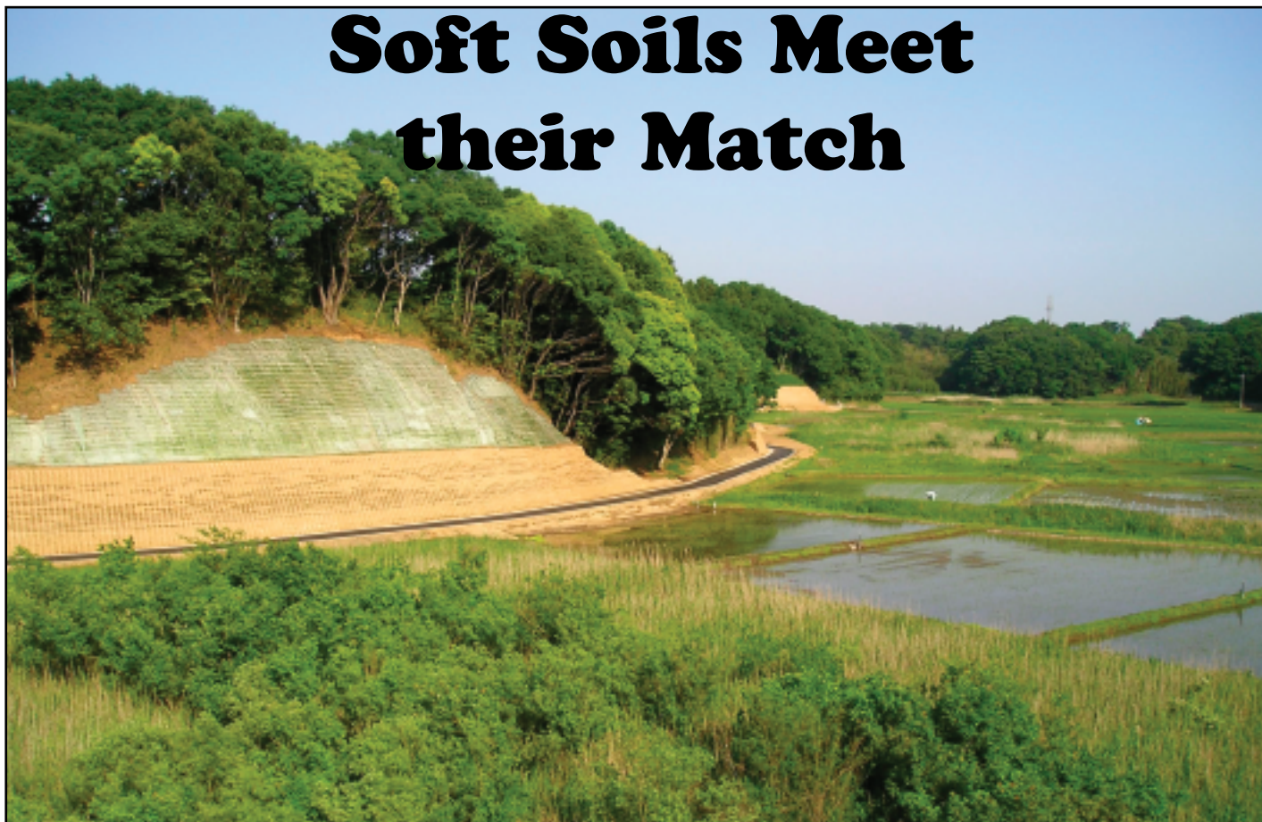
Structurally-stable, light-weight wall structure separates a development area from an extremely soft-soil environment.
