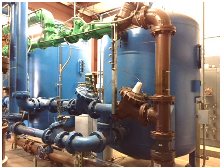
Figure 2-5. Two of the Four Greensand Filters
