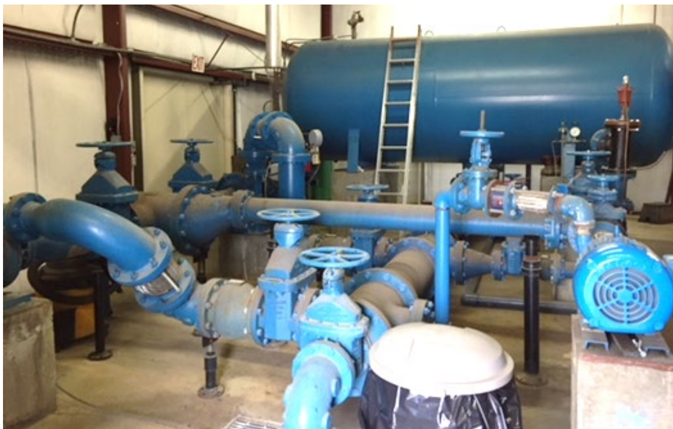
Figure 2-8. Distribution Piping and Pressure Tank
