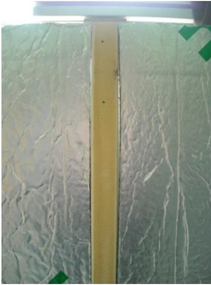
Photo 3 hand cut insulation
