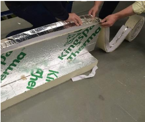
Photo 5 installation of Gapotape
