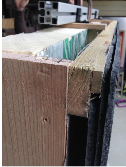
Photo 4 ventilated air cavity
