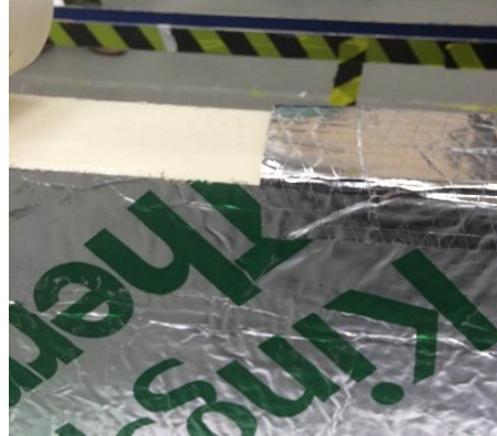
Photo 6 start of the Gapotape application
