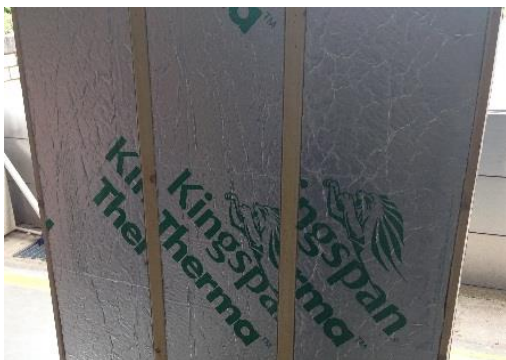
Photo 1 (Kingspan insulation between rafters)
