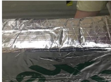
Photo 8 Joint where the ends meet
