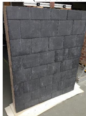
Photo 2 (Tiled outer surface)
