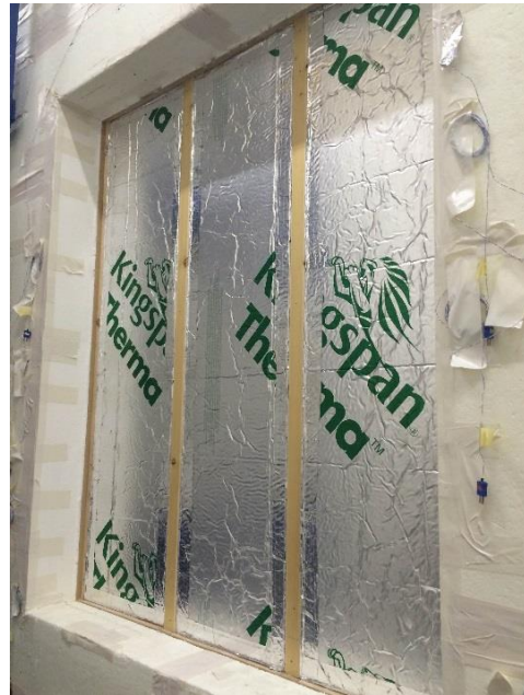
Photo 10 all boards installed
