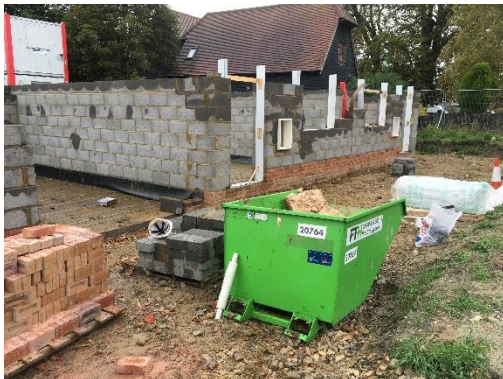
Plot 8 first lift brick & blockwork
