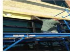
Vapor Barrier being installed over Dens Glass
