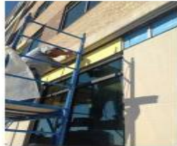
Dens Glass being applied over Hat Channel
