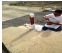
Bollasters on W & N Elevation being prepped and primed for painting
