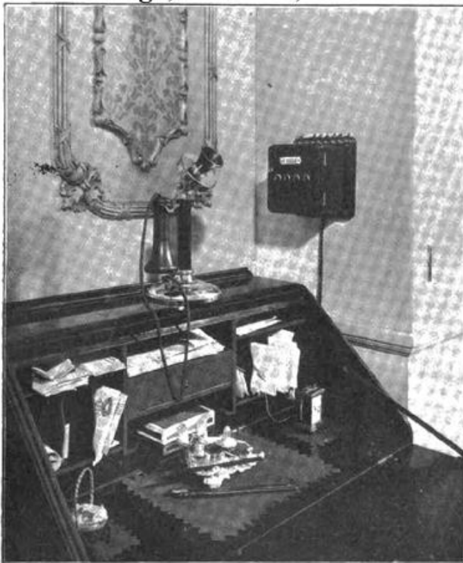
FIG. 6.—SUBSCRIBER'S INTERCOMMUNICATING SET.
