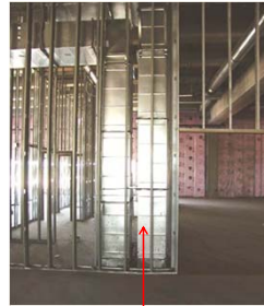
Ductwork penetrating floor
