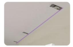
The most difficult part about installing traverse rods is getting the brackets even, level, and straight. A variance of as little as a 1/8" can prevent you from being able to install your rod correctly. Choose your desired location to mount brackets and mark with a pencil. Make sure that all brackets are aligned evenly across and verify using a level. Brackets should be positioned every 3-4 FT. Never, under any circumstances, use hollow anchors with brackets.
