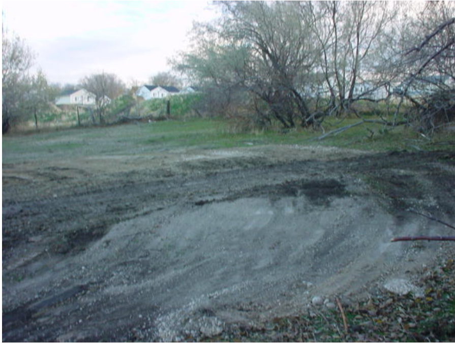
Figure 5: Test pit 4 location backfilled viewing southeast.
