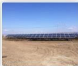
Reci, Covasna, RO 2,133 MW
