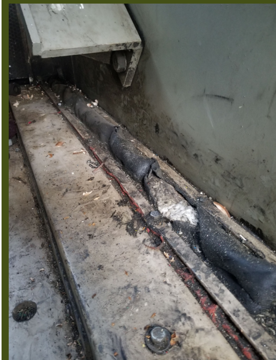
Before - Load Compartment Floor
