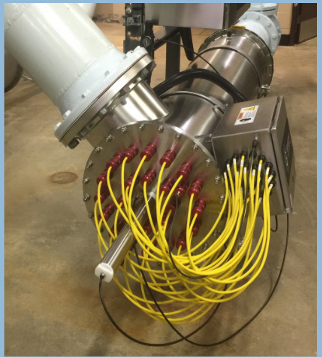
New 316L chamber holds 24 UV lamps
