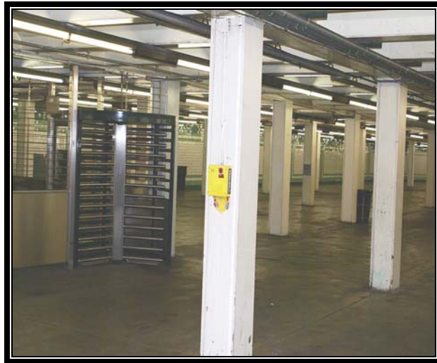
Figure 16. New box with no backing.
