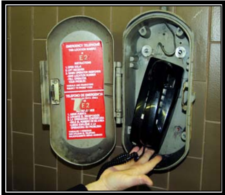
Figure 7. Damaged phone
