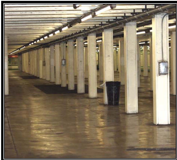
Figure 15. Recently installed call box is mounted on the rear of the first pole. Note that the pole is not marked in any way whatsoever.
