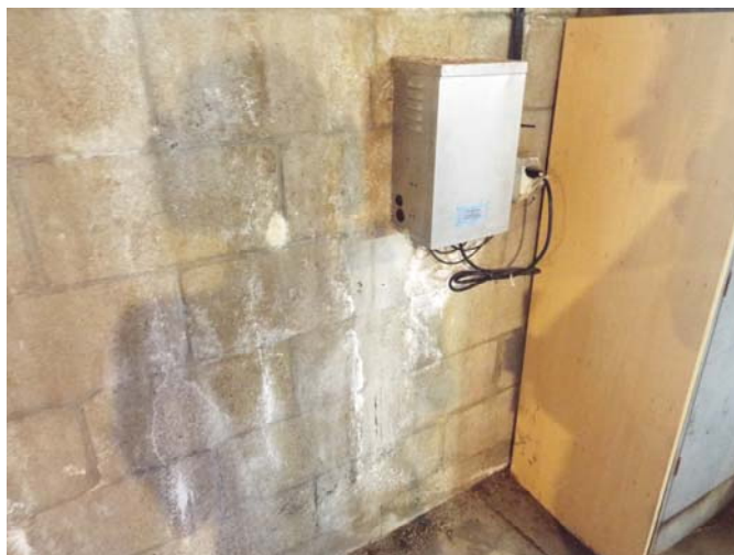
Efflorescence observed at block wall.
