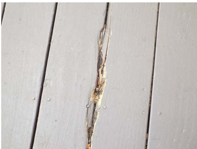
Isolated area of deteriorated wood.
