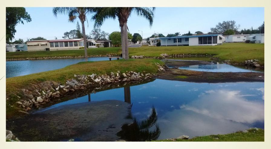
Silt build up in this pond adds to continued flooding on Moog Road and Jarvis Street. Pond to be dredged in order to allow proper water flow.
