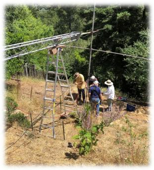
The disassembly of the antenna sections required a series of rotations and section removals. Ultimately the entire antenna mast and rotor were removed prior to disassembling the tower itself. The tower was disassembled from the bottom section to the top, section by section. The remainder of the tower was slid toward the house as each section was removed.
