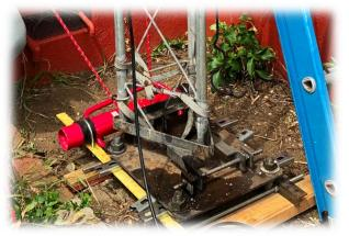
(mounted with four bolts to the concrete footing) and a triangular steel structure at the bottom of the tower. This piece was attached to
