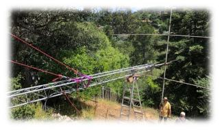
The lowering took place by removing a pin at the rear of the base to release the tower for pivoting. The weight of the tower was now supported by the pivot at the base and by the lowering rope from above. Once the tower had cleared a roof obstruction, it was lowered toward a ladder set up to support the tower for disassembly.
