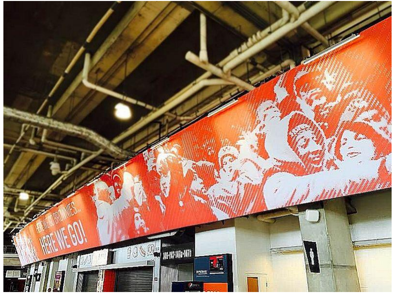
TS32 - Cleveland Browns Stadium- Food court Banner stretched on a 310' by 13' existing steel frame.
