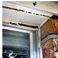
6. While cleaning the windows, check the caulking at joints around doors and windows, where wiring and pipes enter the home, and where different building materials meet can help keep water, insects, and hot air out. Also, sealing joints where concrete patios or walkways, and driveways meet the home can help prevent water entry.
