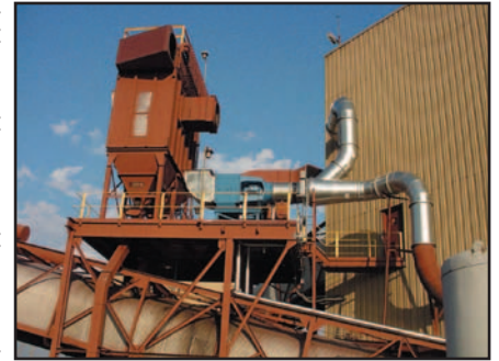
Engart Unit replacing dry bag house collector
