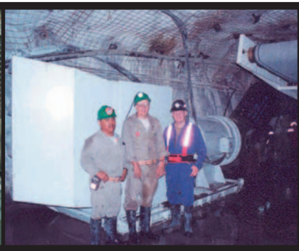
Underground face ventilation
