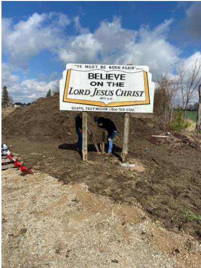
Palmerston, ON reinstalled
