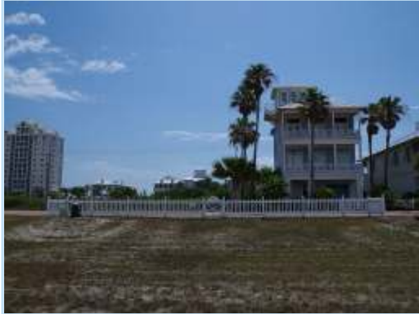
8405 Main St view from lot facing east
