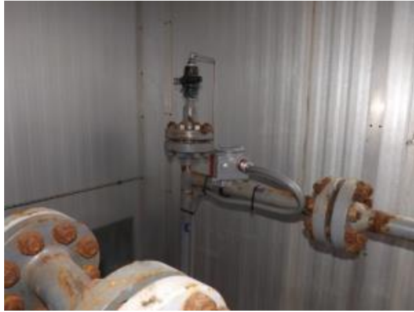
IMELDA unit mounted to pipeline and plumbed to ball valve
