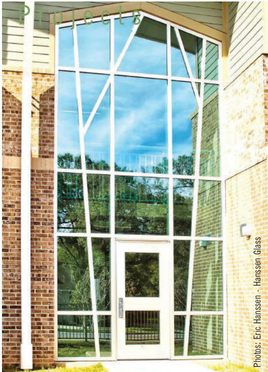
An artistic muntin pattern in the curtainwall elevations was a unique glazing design element.
