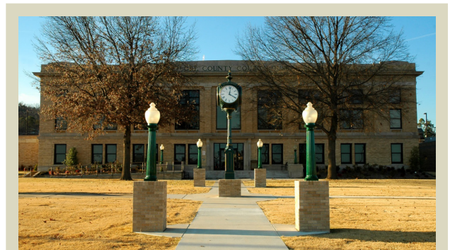
LeFlore County Courthouse, Poteau
