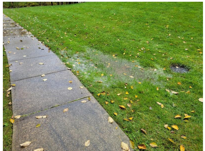
16. View of a low area in the landscape adjacent to a common walk. Note the ponding water.
