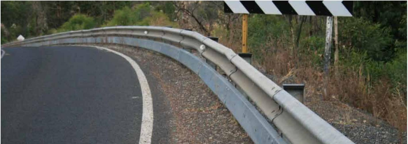
*An example of additional protection added to a barrier to allow a rider to slide along the barrier and prevent colliding with a post in a crash.*
