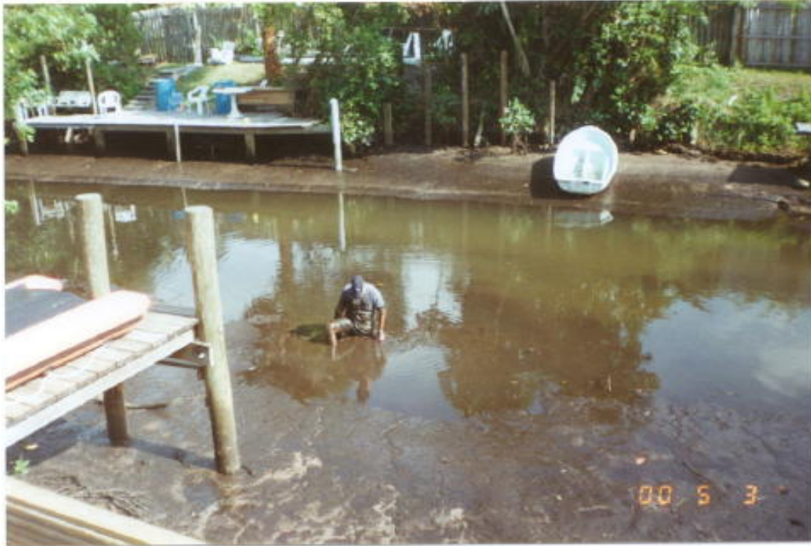
Jones Creek Restoration (Before)
