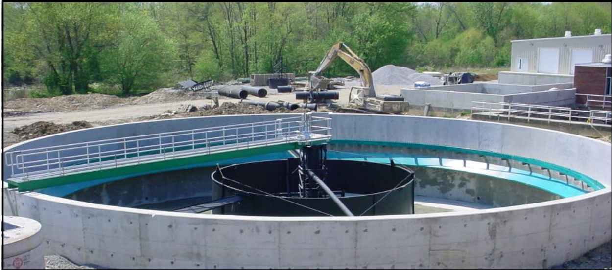
Stamford Baffle at Moorehead, KY with 1'6" long baffle brackets with right angle upper bracket for algae sweep.
