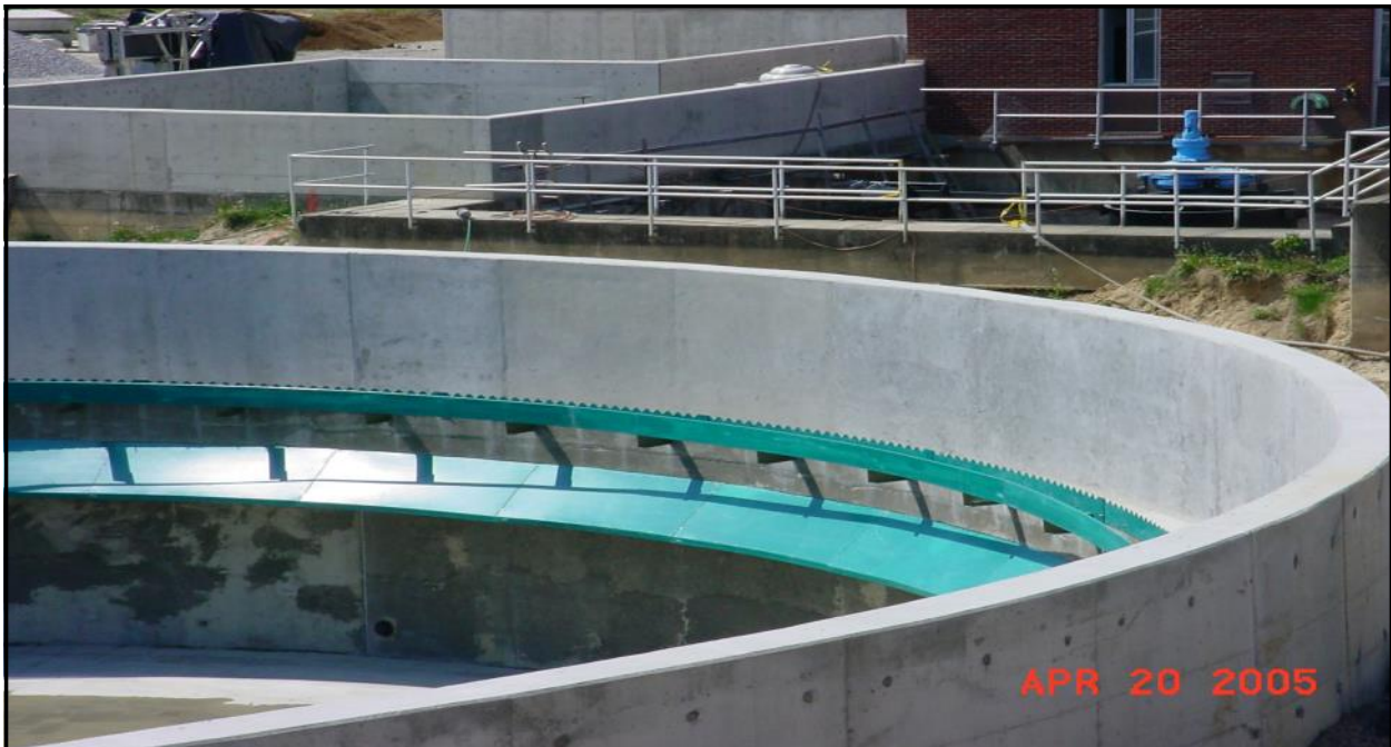
Closer view of above. All components are pultruded fiberglass shapes with superior strength, corrosion resistance, and UV resistance to molded or hand laid-up materials.
