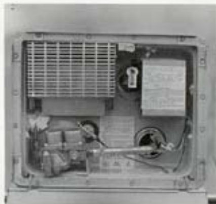
Water Heater Outside Access Compartment
