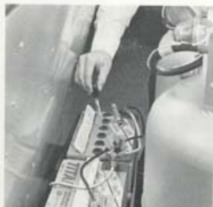
Battery Hydrometer Check
