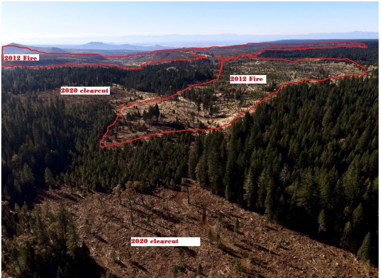
Figure 49. The Reynolds Flat THP was filed in 2012, but all of its units were not cut; some of the units were interspersed with the area burned in the 2012 Ponderosa fire. In the summer of 2020, around the time fires were starting all over California, the Reynolds units were cut, adding more open, dry land to the watershed which fails to dissipate incoming solar radiation.
