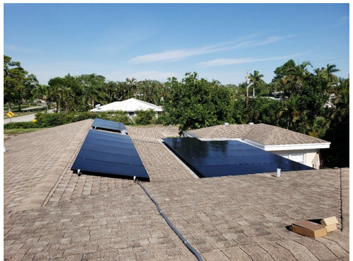
Solar Panels Installed
